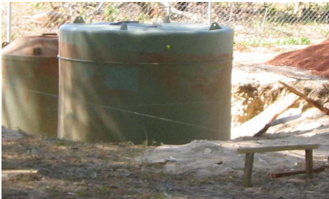
With a good bore found, the tanks are set in place.
