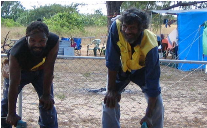
Aide and Pungi building the platforms for tourists tents.
